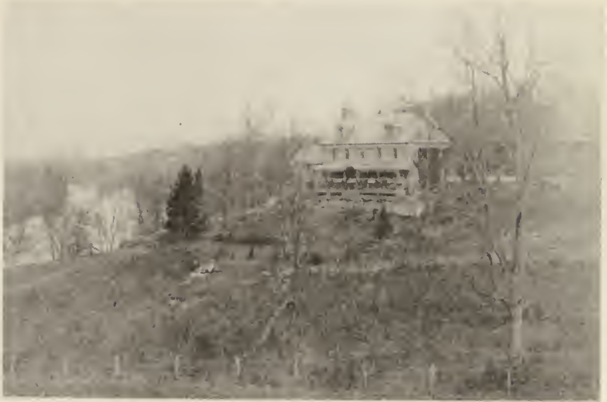
Figure 52. South and east elevations of the main house, believed to date to the 1890s showing the porch under construction. (Mill Grove Files, Audubon, PA.)
